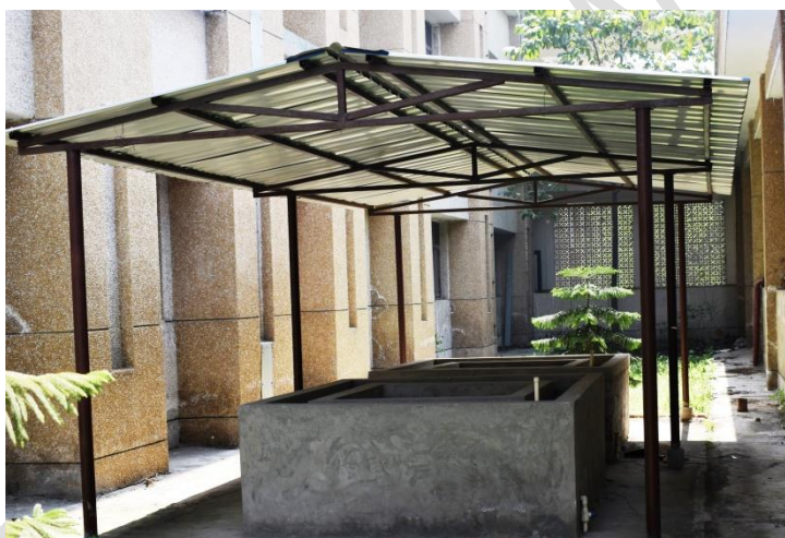
Picture 1: Zero Energy Cool Chamber
