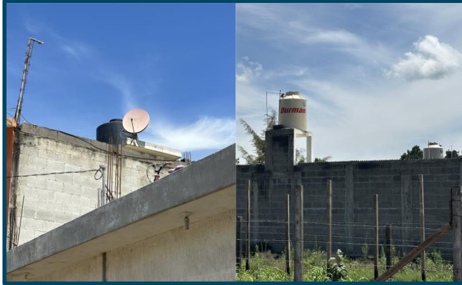
Figure 1. The water tank on the ceiling of Guatemala households
